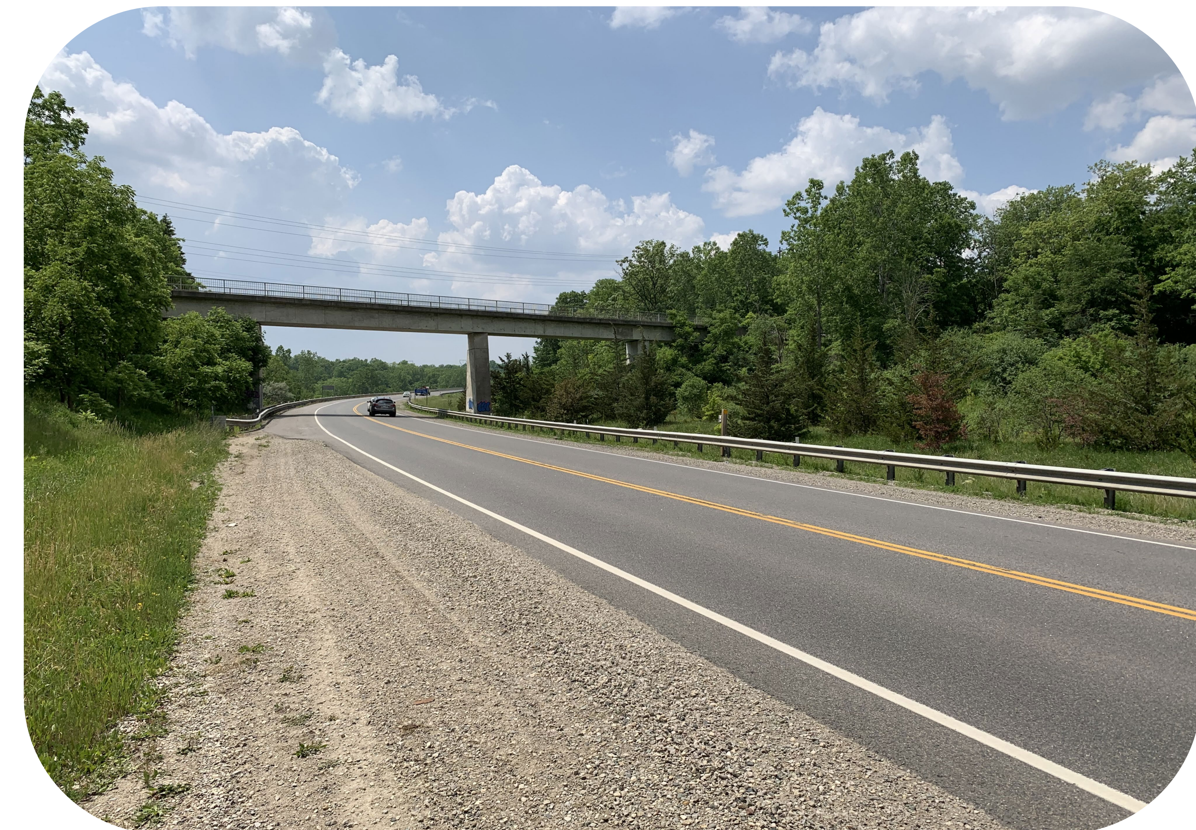
Highway 3 east of CNR Subway looking west.
